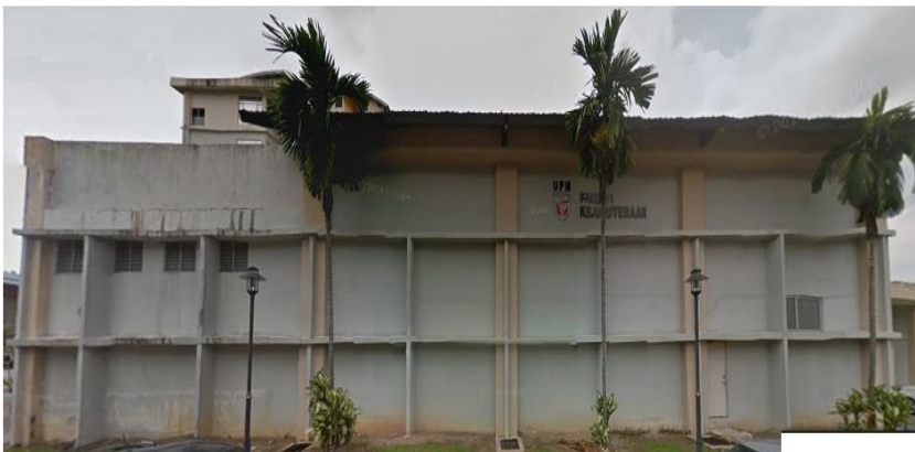
Figure 3. Auditorium Faculty of Engineering UPM
